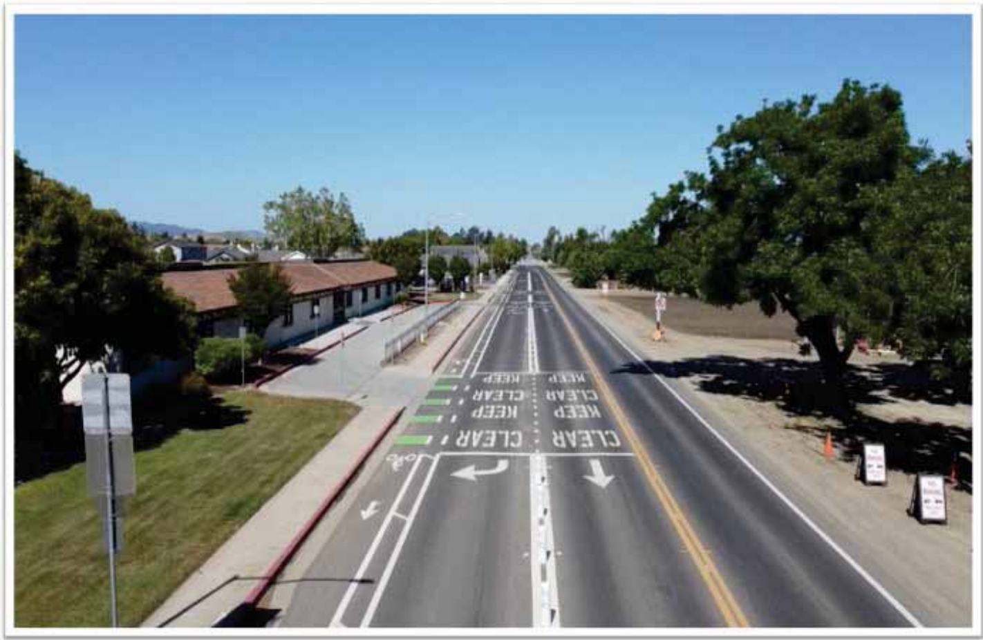
A Measure G funded project on Santa Ana Road in the City of Hollister.
