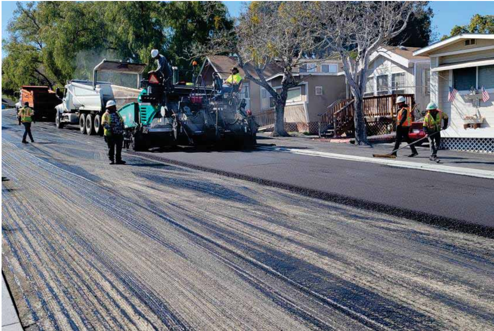
The Measure G funded pavement milling and overlay of Church Street in the City of San Juan Bautista.
