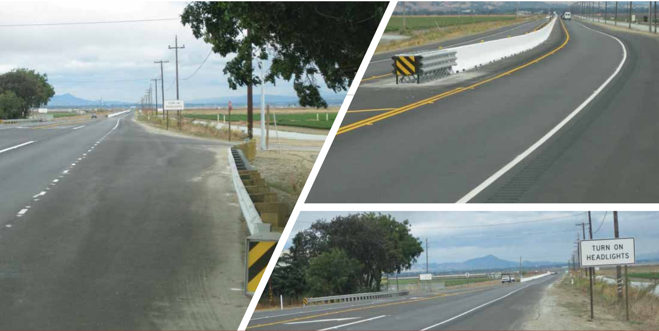
SR 25 Safety Enhancement Project – Constructed 2009
