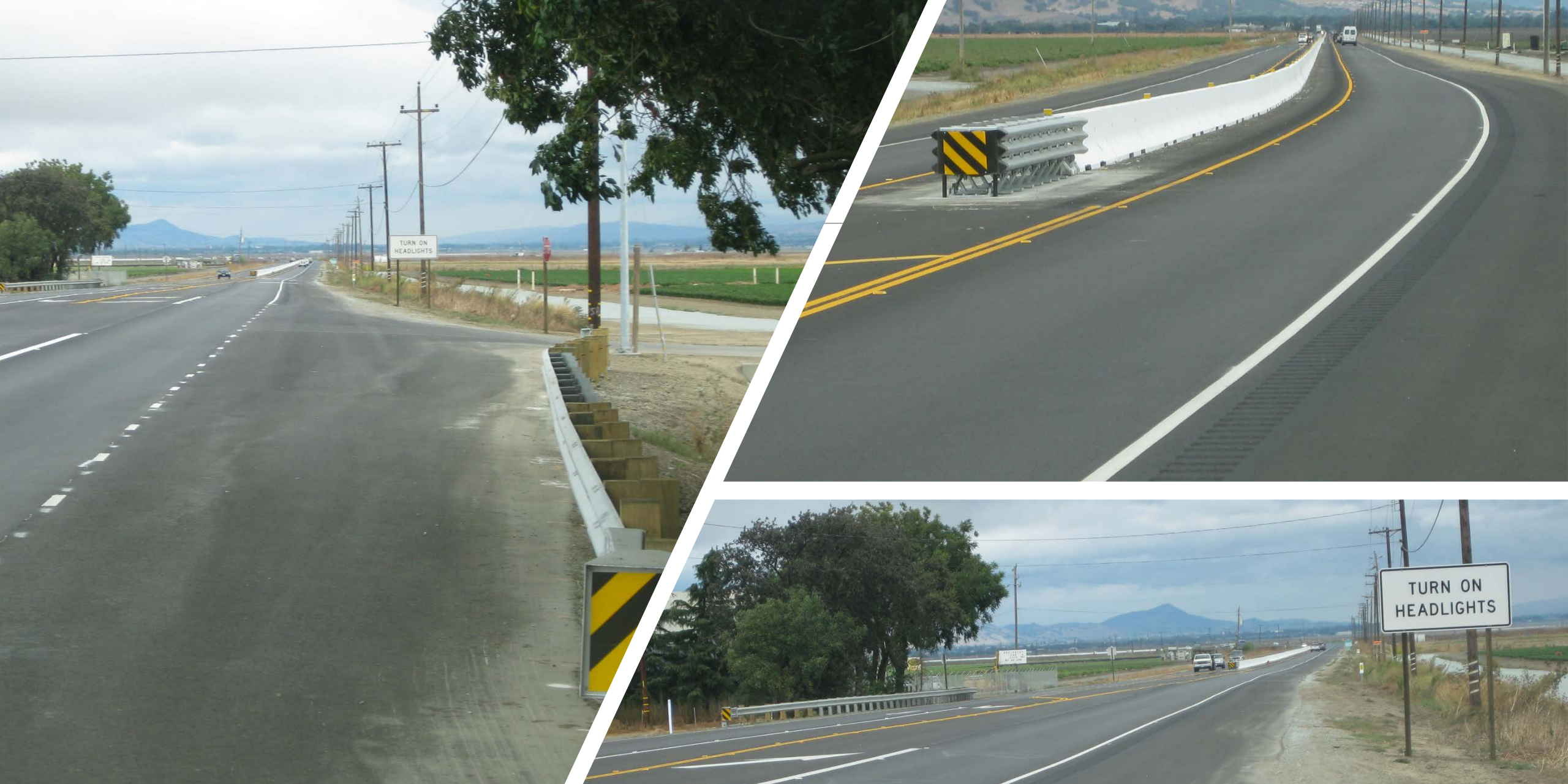
SR 25 Safety Enhancement Project – Constructed 2009
