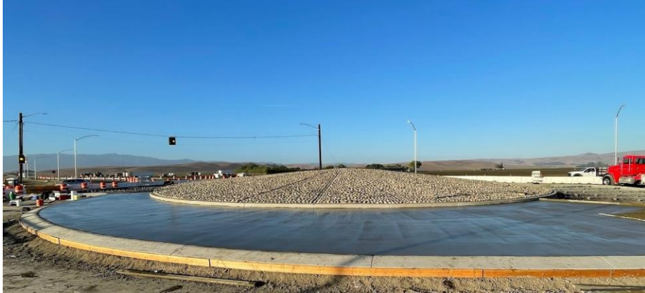
Construction on SR 156/25 Turbo Roundabout
