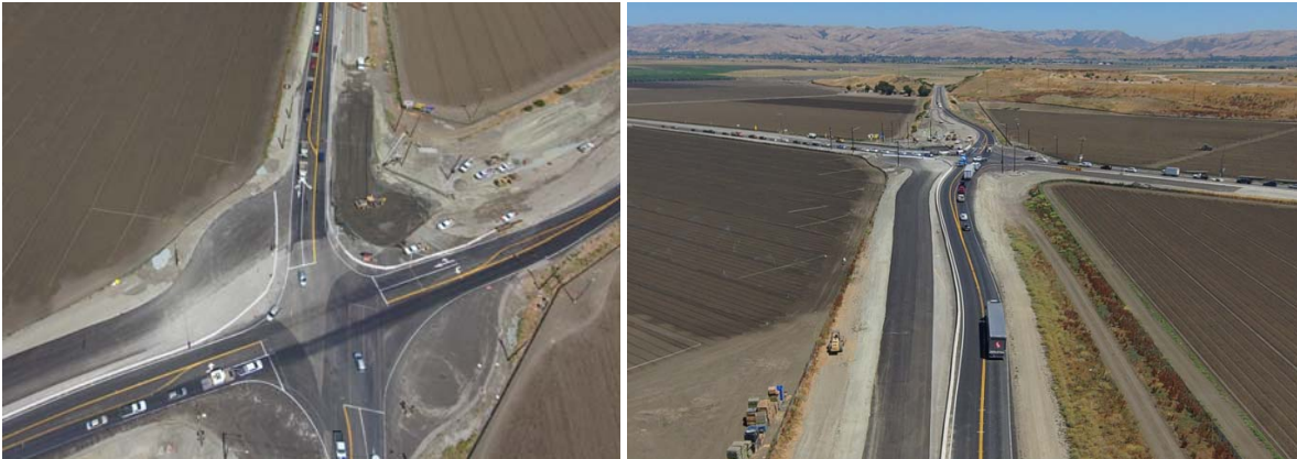
Construction on SR 156/25 Turbo Roundabout
