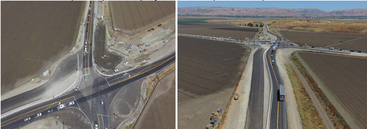
Construction on SR 156/25 Turbo Roundabout
