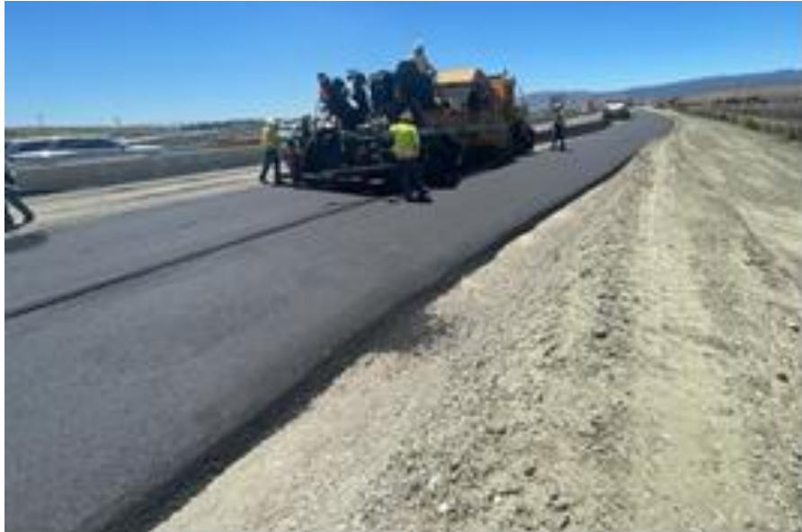
Construction on SR 156/25 Turbo Roundabout
