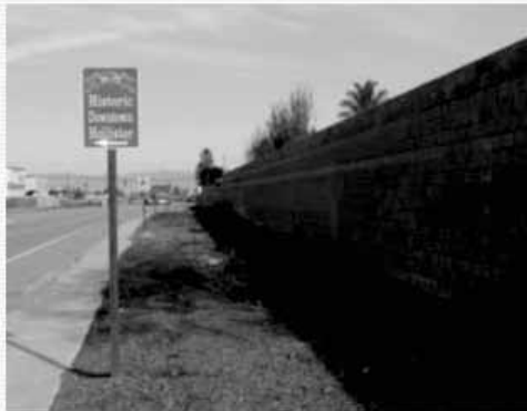
Typical Existing Rt. 25 roadside and soundwall
