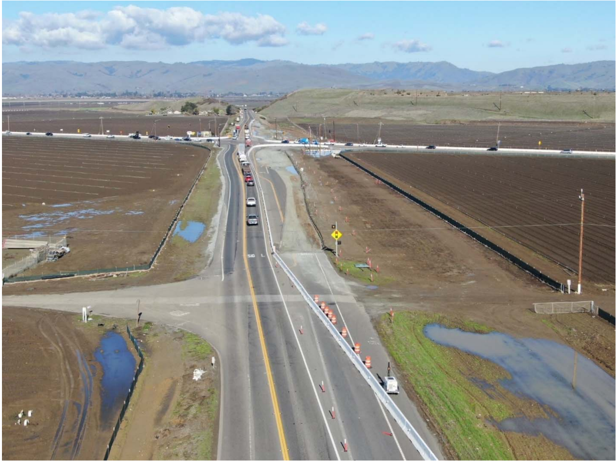
Aerial photo of Roundabout construction at Hwy. 25 and 156, mid-December 2022.
