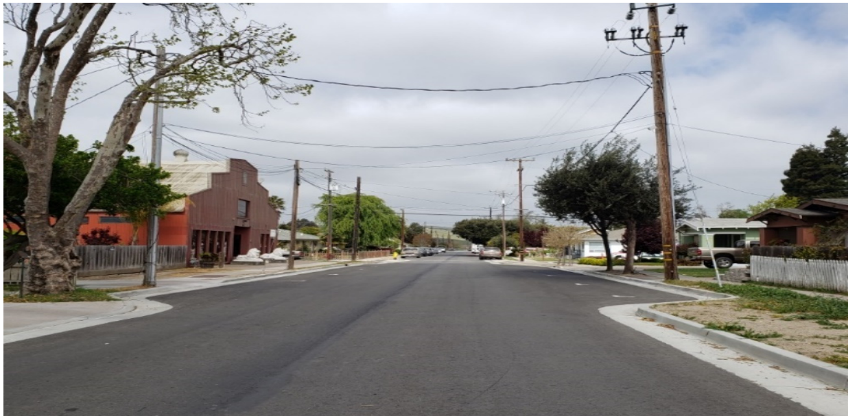
Figure 1-4: First project completed under Measure G, Third Street Pavement Resurfacing Project, City of San Juan Bautista
