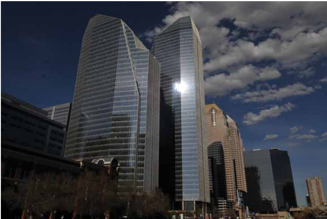
Figure 13: Solas Glare Catalogue Image ( 158 \text{ W}/\text{m}^2 ) at a similar irradiance level to those expected at the Project
