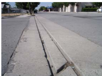
Examples of bicycle unfriendly slot drain
