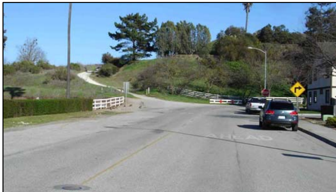
Looking east from Buena Vista Road to the future Buena Vista Road extension to North Street/McCray Street.
