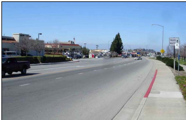
Looking north on Highway 25/Airline Highway, between Sunnyslope Road and Sunset Drive.
