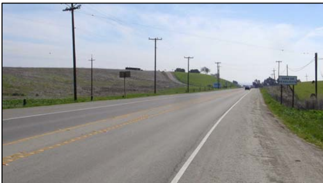
Highway 25, south of Highway 156, looking south.
