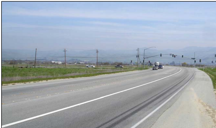
Looking east on Highway 156, towards San Felipe Road.
